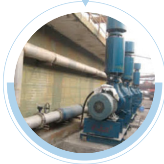
焦化厂污水 Coking Wastewater
