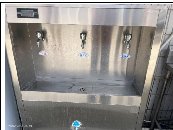
NC-7.9 No high temperature warning sign posted nearby the drinking water device.
